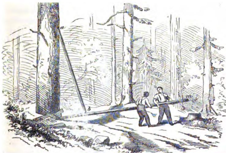
Fig. 144.—Throwing a stem with levers.
